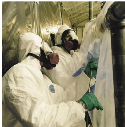
Trainees in a recent Lead Worker Certification class practice encapsulating simulated harmful materials.
